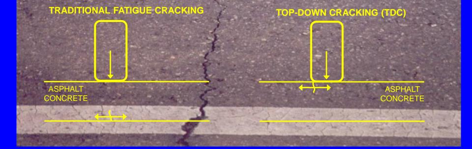
TOP-DOWN CRACKING OF ASPHALT CONCRETE IS NOT GENERALLY CONSIDERED IN CURRENT ASPHALT DESIGN PROCEDURES IT IS NOW BEING CONSIDERED FOR LONG-LIFE ASPHALT PAVEMENTS
